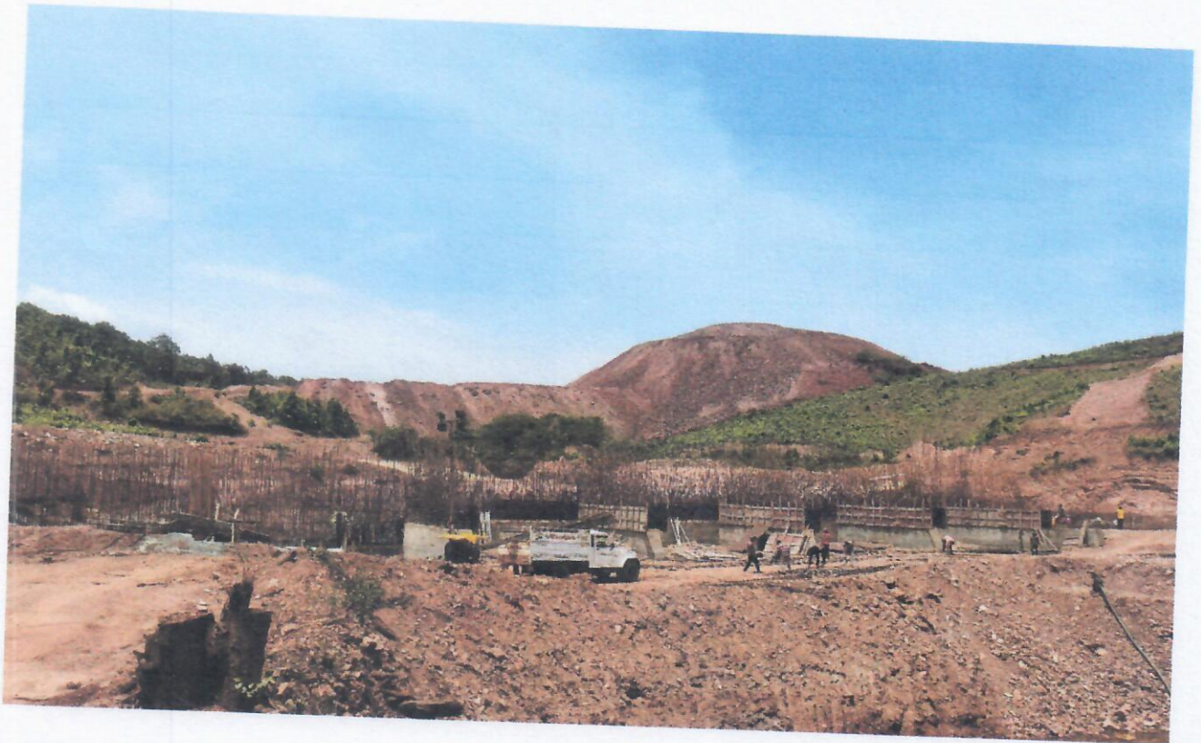
Exhibit- Retaining wall at the toe sub-grade dump
